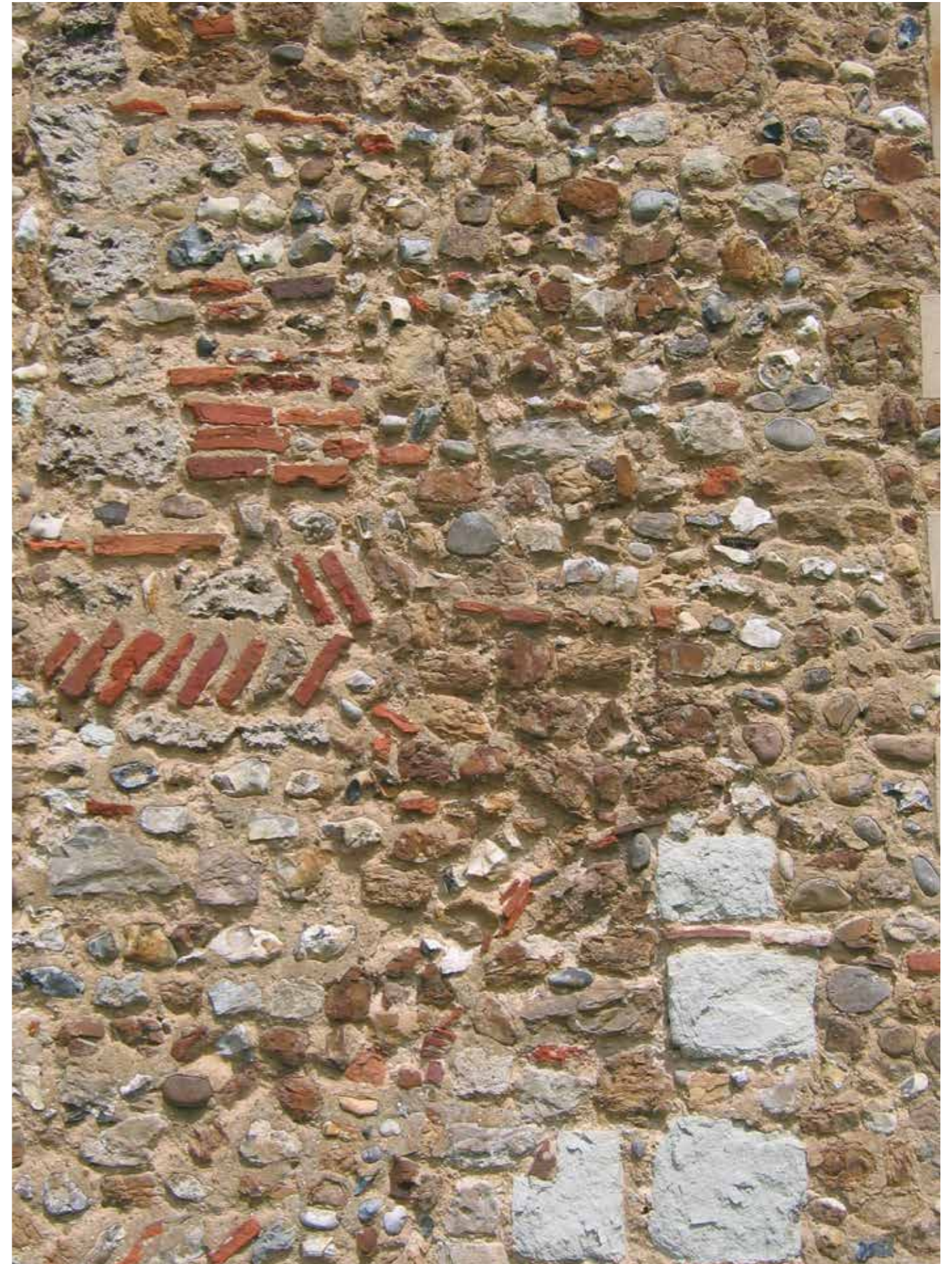
Old church wall built of rubble laid to courses. It includes Roman brick, peg tile, flint, septaria, tufa, Ragstone and Reigate stone.
