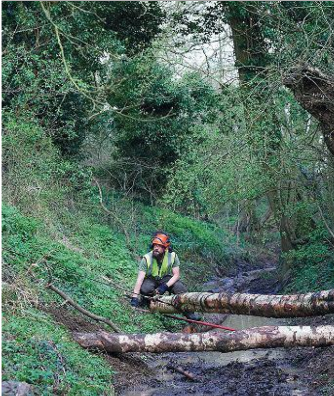
Figure 10: Evidence to action case study of leaky dams in Essex. Images from Floods Team at ECC.
