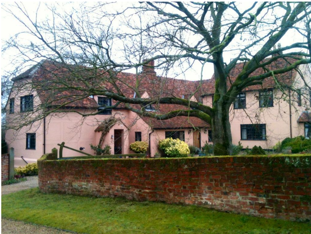
Fig. 3 View of Chamberlayne Farmhouse, Clavering
